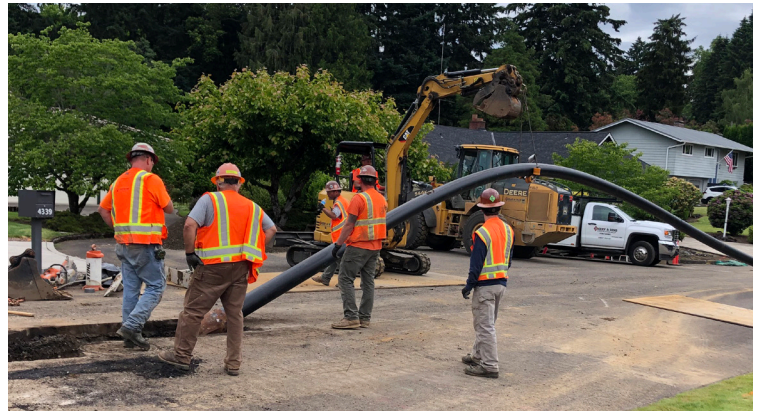
OLWS SE Old Orchard Court Water Line Improvements
